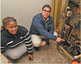
Time to cut the cord: As illegal electricity connections from Monwabisi Zone 4 were putting the operation of the Swartklip Road sewer pump in danger, the City had to step in to protect its infrastructure and the community's safety. Pictured inspecting the pump station are Lerato Mbuzwa, regional pump station manager, and Cllr Zahid Badroodien, Mayoral Committee member for Water and Sanitation.
